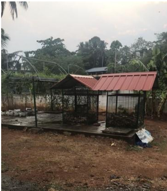
Aero bins for Minimal Wastes and no leachate management
