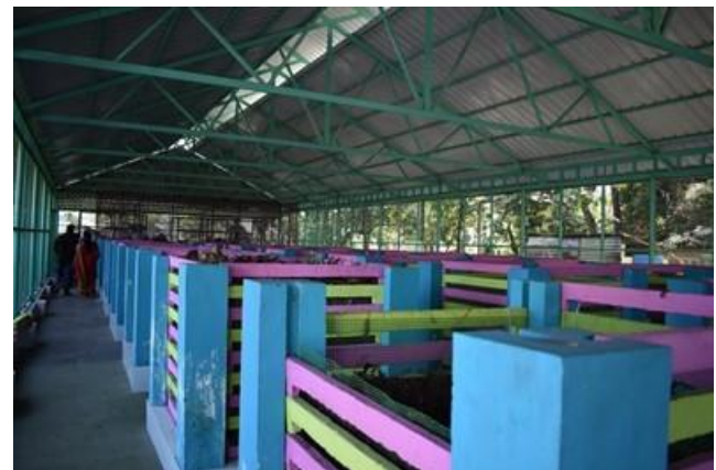
Aero bins for Minimal Wastes and no leachate management
